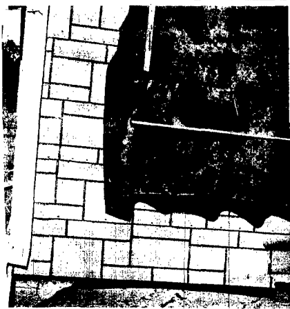
A GAS EXPLOSION at Dixon last week knocked the house of Bill Kraemer off its foundation a little bit. One corner is shown above. Note that the house is a little to the right of the foundation, and that is a big crack in the lower left corner. Windows blown out are covered as shown until repairs can be made.
